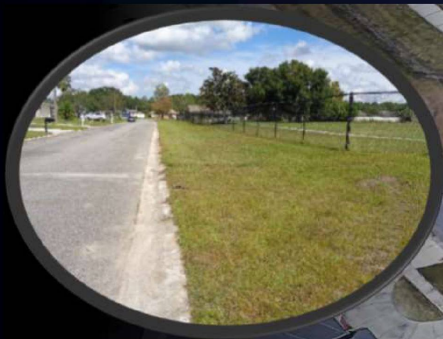
Valley Gutter at Babbitt Ave.
